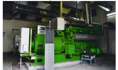
Combined heat and power system producing electricity and steam
